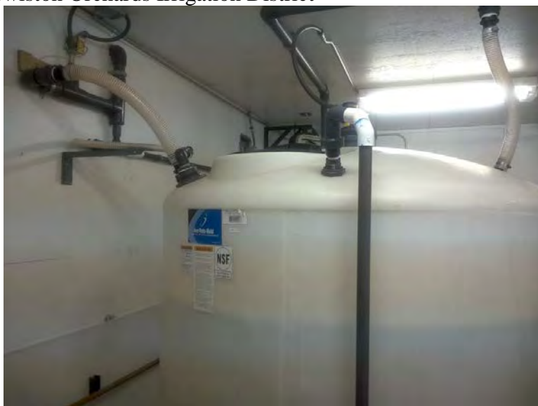
Photograph 18: Well #4 Chlorination Daytank
