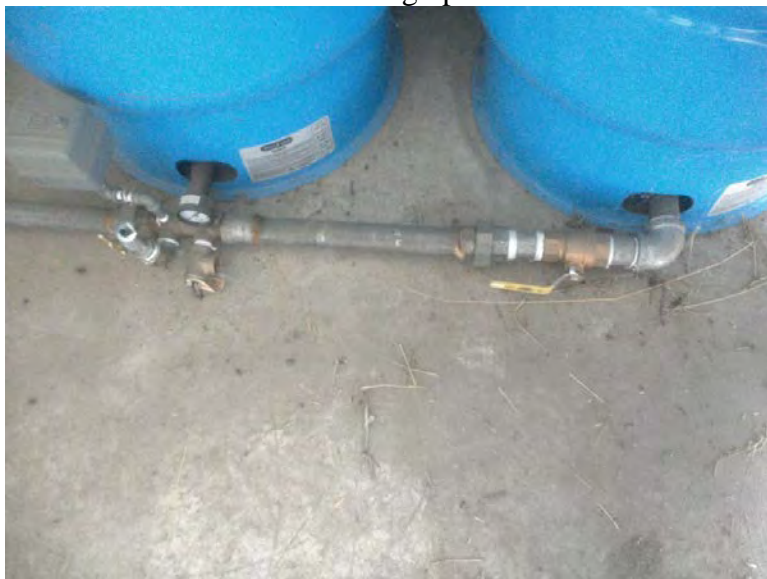
Photograph 53: Filter Plant Hydro Tanks Isolation Valve
