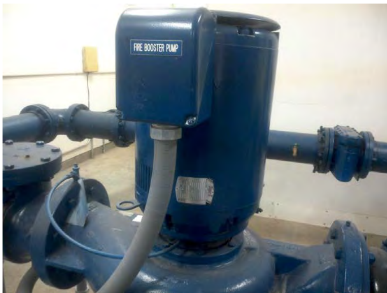
Photograph 32: Lutes Booster Station Fire Pump
