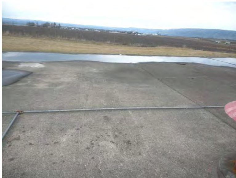
Photograph 44: Filter Plant Reservoir Standing Water
