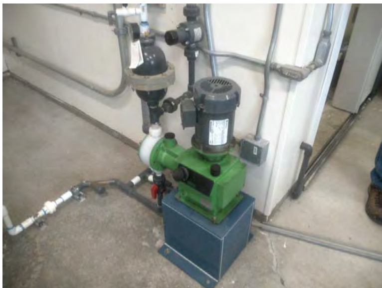
Photograph 27: Well #3 Chlorination
