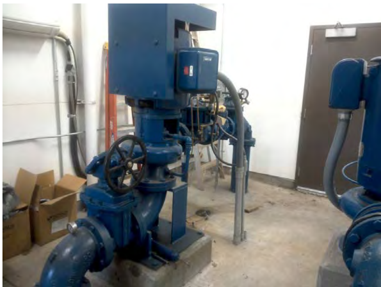
Photograph 31: Lutes Booster Station Transfer Pump
