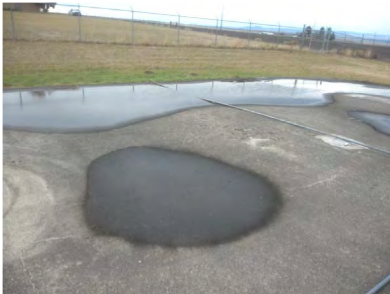
Photograph 43: Filter Plant Reservoir Standing Water
