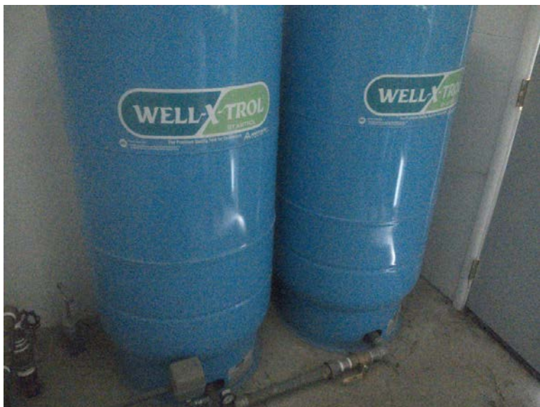
Photograph 52: Filter Plant Hydro Tanks
