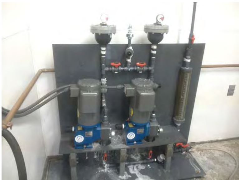
Photograph 19: Well #4 Chlorination
