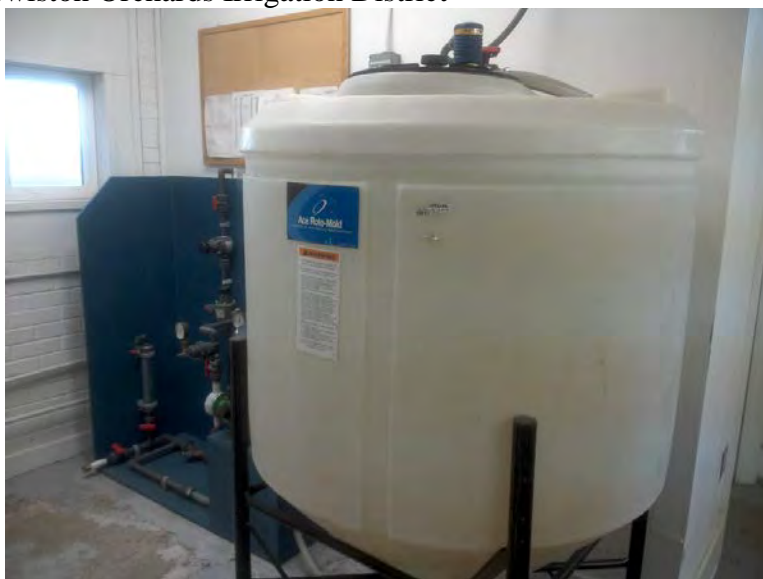
Photograph 38: Well #2 Chlorination Daytank
