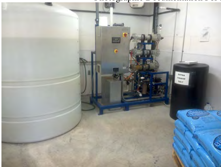
Photograph 17: Well #4 Chlorination
