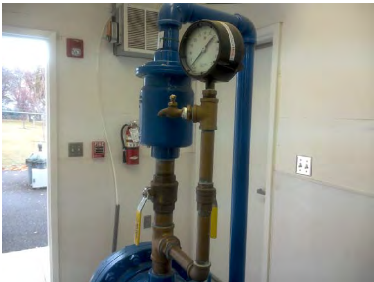
Photograph 15: Well #4 Sample Tap and Pressure Gauge
