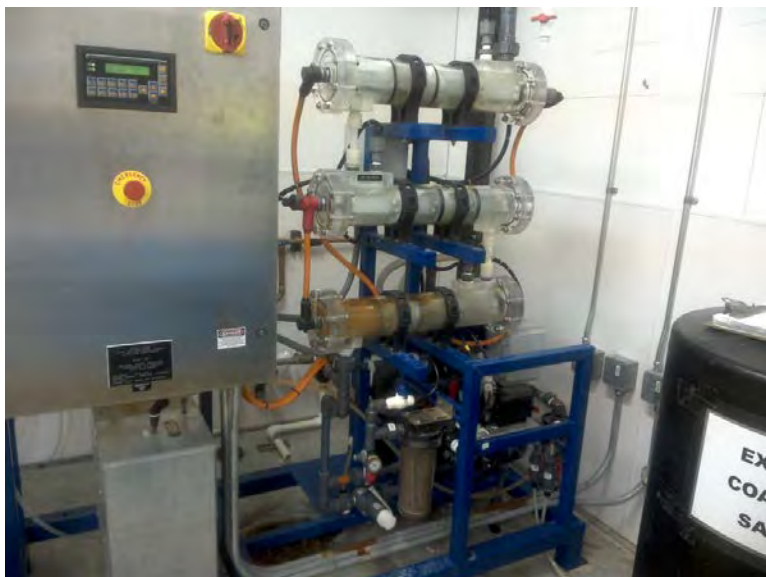
Photograph 20: Well #4 Chlorination
